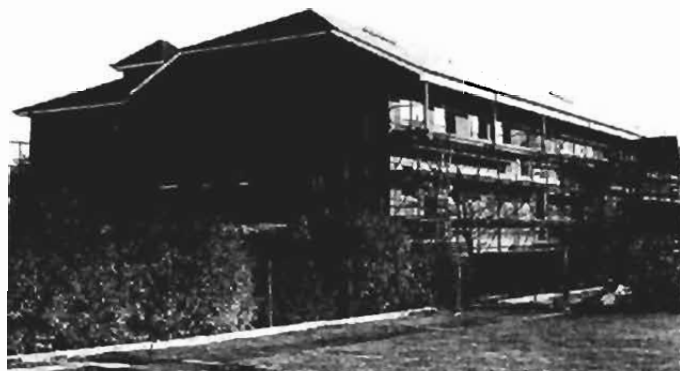
Conway Building nears completion
